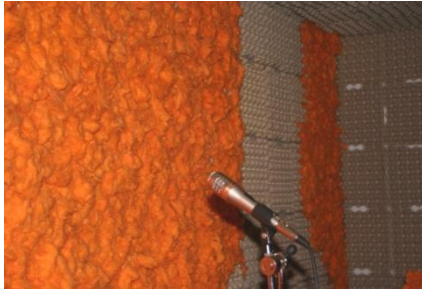
Figure 2. Image of the anechoic room under construction.
